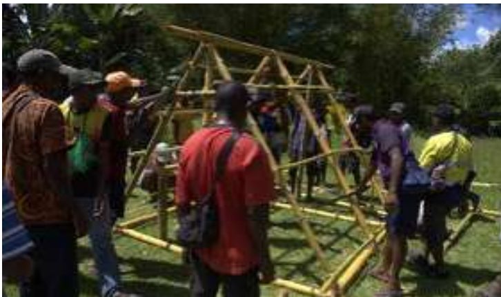
Photo 1. Training participants are building a solar dryer to dry grated cassava and sweet potato for fish feed production.
